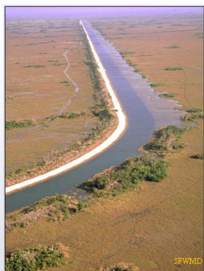
Figure 3: C-111 canal site TS/PH-4 after levee removal.
