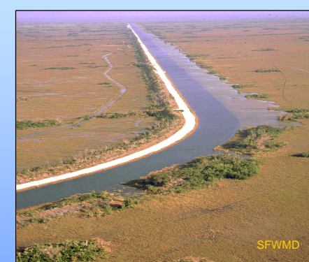
Figure 3: C-111 canal site TS/PH-4 after levee removal.
